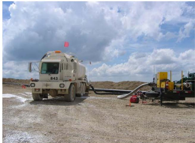
**Figure 4:** Slurry transport truck offloading slaked lime during down-hole injection stage.
